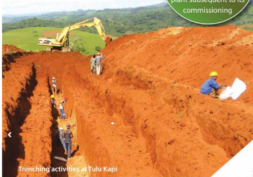
Trenching activities at Tulu Kapi
